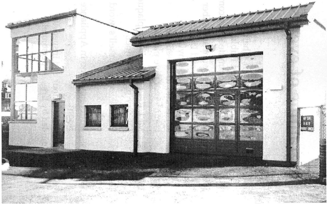
Langholm's new Fire Station — opened Friday, 11th October, 1996
